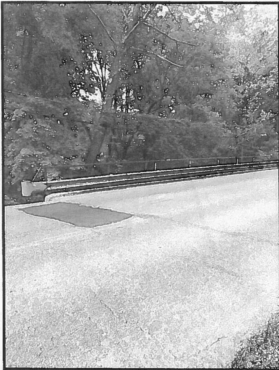
East side of bridge (site photo)
